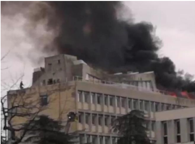
17-Jan-2019 (Tribune.com.pk) Kebakaran besar di atap sebuah universitas di Lyon, 1 luka berat / Large fire on roof top of a university in Lyon, 1 injury.
